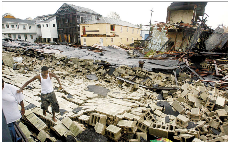
Lester Thomas, 12, of New Orleans steps through rubble of a building on Terpsichore Street that was destroyed Monday by Hurricane Katrina. He said he rode out the storm in a small house next door with his grandmother and 13 other relatives.
